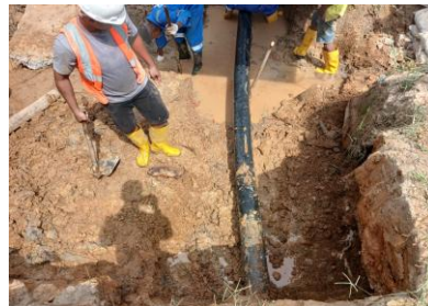
Figure 3. Top View of the Field Team Conducting Excavation and Pipeline Inspection at KP.03+500
