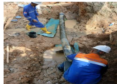
Figure 4. PT XYZ Technical Personnel Conducting Direct Inspection of the Pipeline and Coating Condition at the Inspection Site
