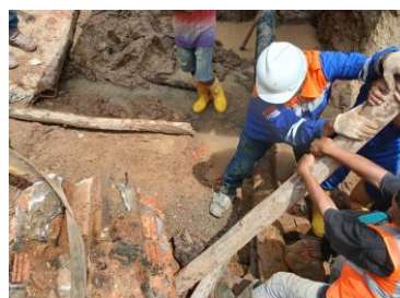
Figure 5. Soil Stabilization and Structural Support Activities in the Pipeline Excavation Area at KP.03+500
